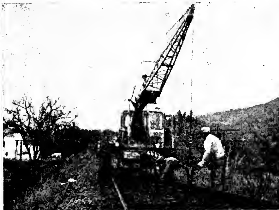
LAYING STANDARD RAIL
